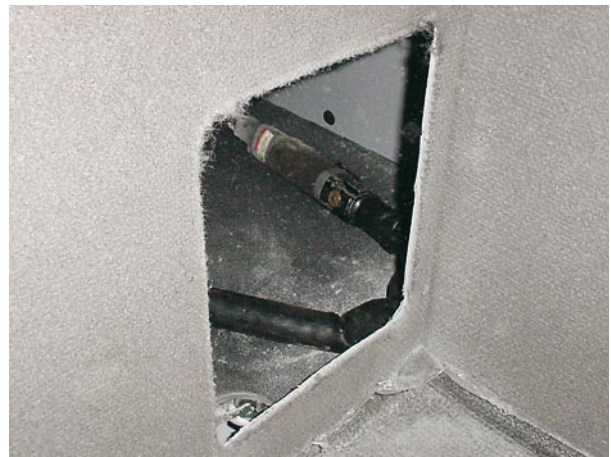
Figure 9 - Return air vent hole cut
